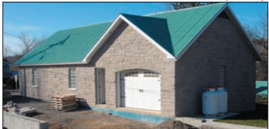
South view of the workshop.
