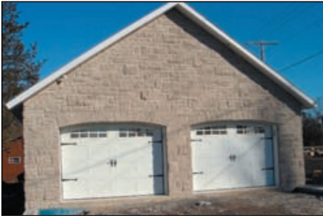
West view of the garage.
